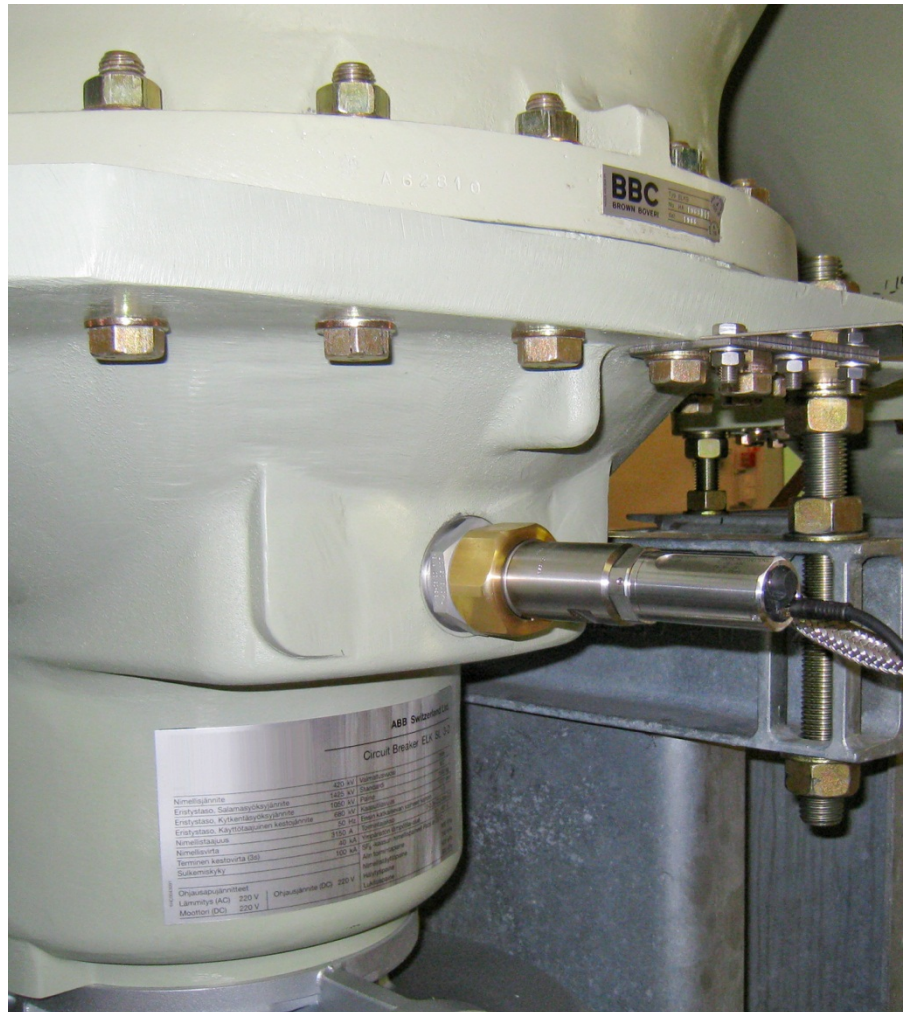
Figure 7 Indoor Installation in a Circuit Breaker
